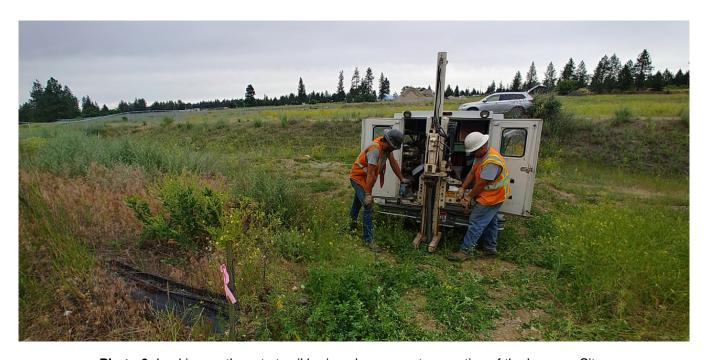
Photo 6: Looking northwest at soil boring along a western portion of the berm on Site.
